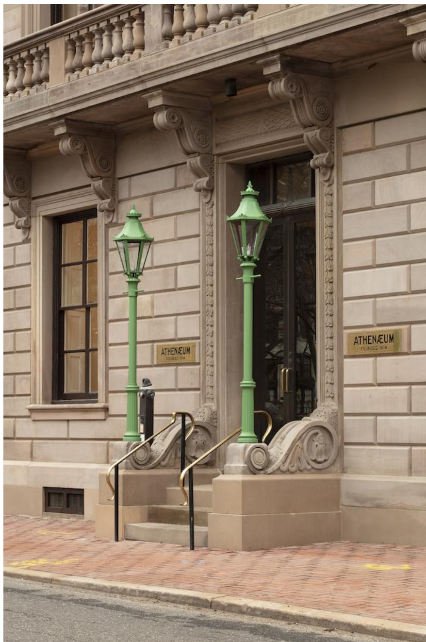
The Athenaeum's west entrance after exterior renovations. | Photo: Photo: Joseph E.B. Elliott via The Athenaeum of Philadelphia
