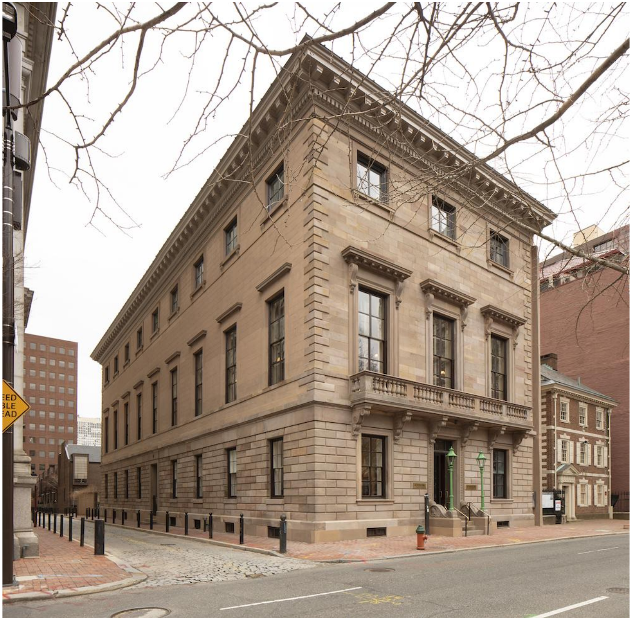
The Athenaeum of Philadelphia at 219 S. 6th Street after recent exterior renovations. | Photo: Joseph E.B. Elliott via The Athenaeum of Philadelphia
